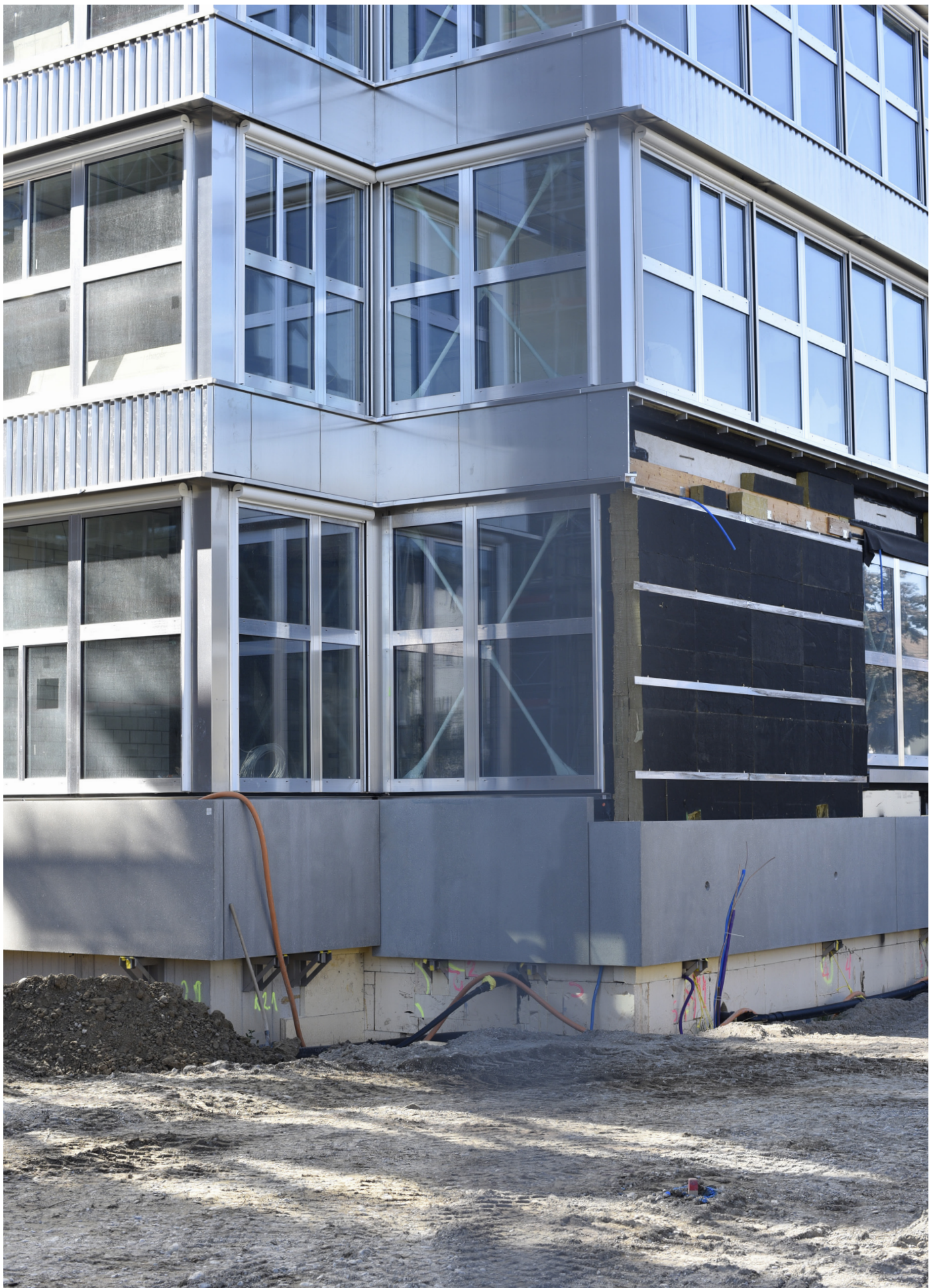
36: Installed Insulation Panels Source: Own
