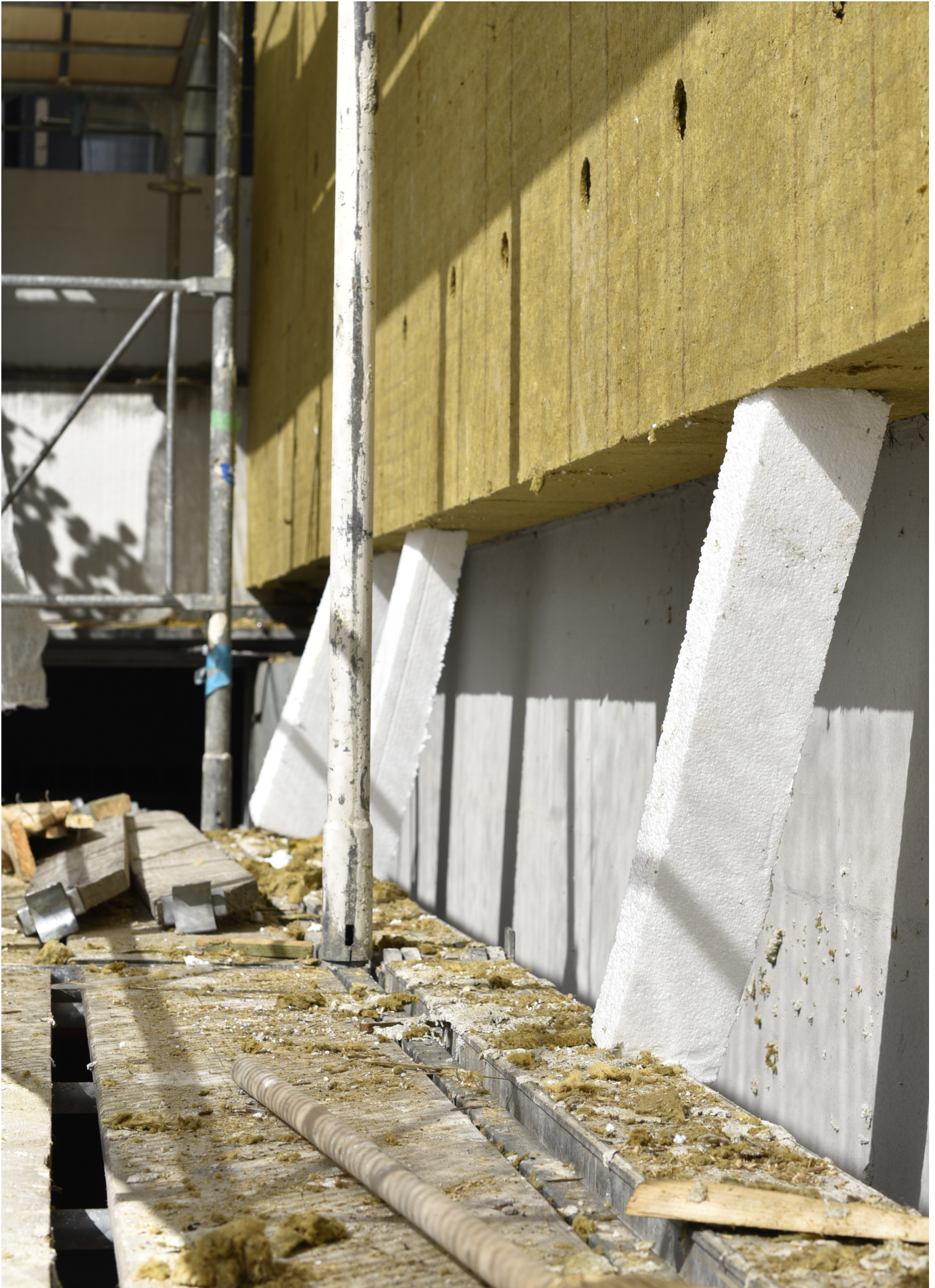
32: Insulation Doubling for Retrofitting Source: Own
